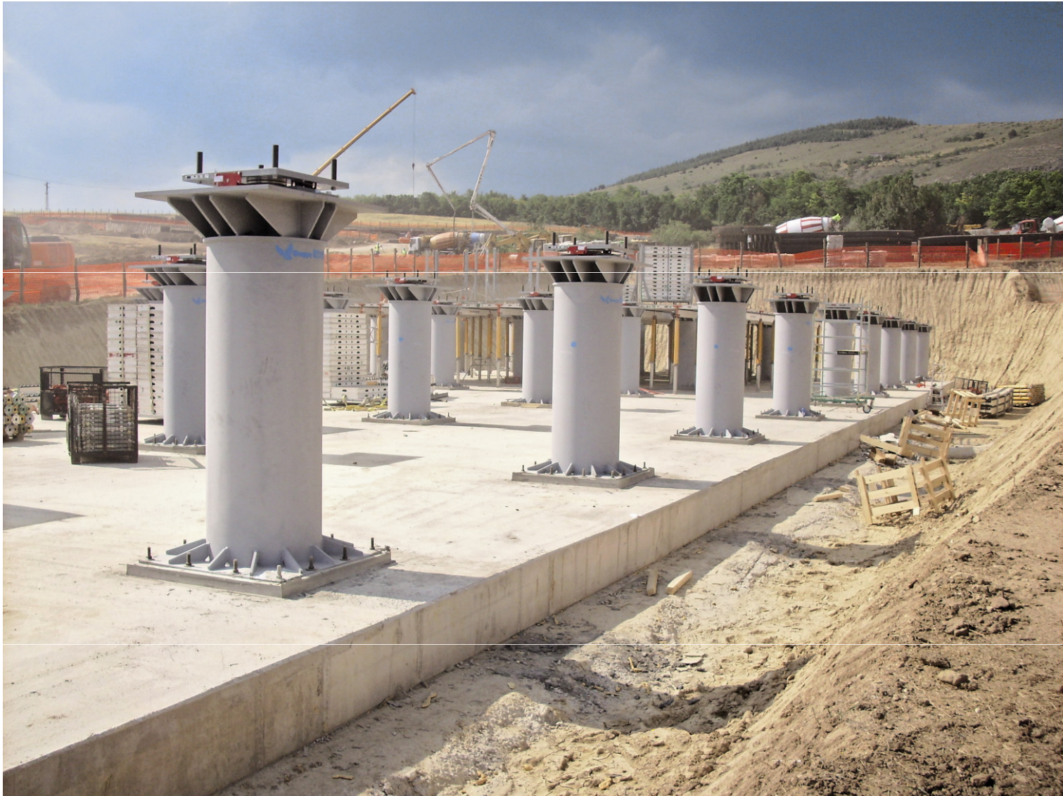
The sliding pendulum isolators on top of the 40 steel columns supporting the concrete slab
