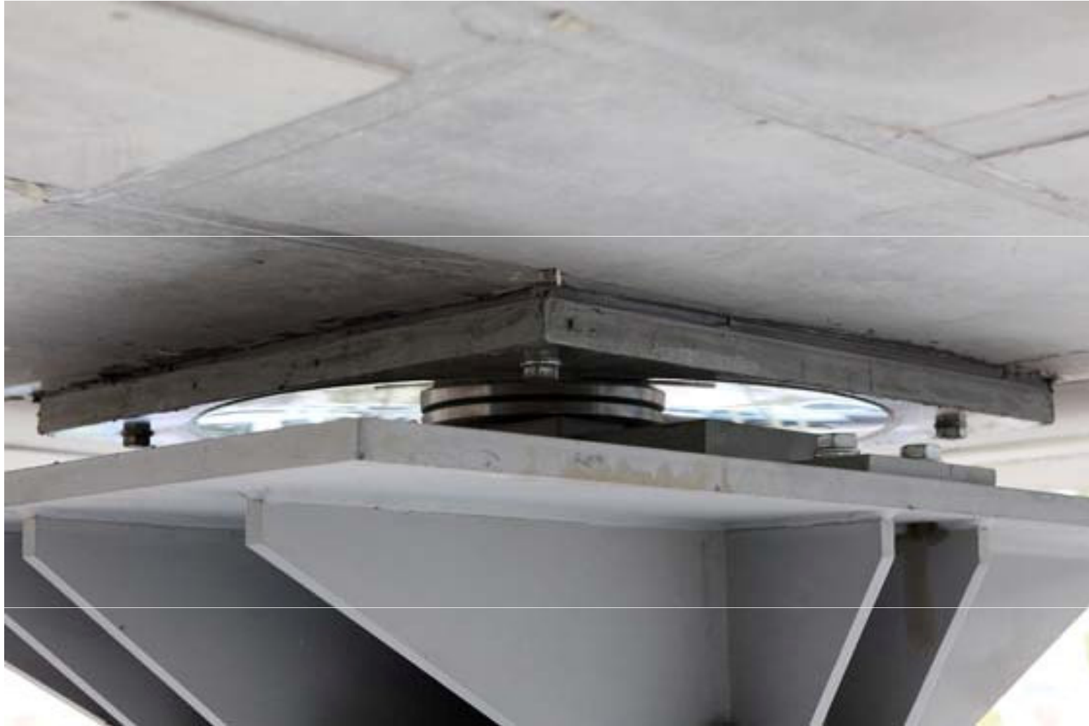
Detail of an isolator on top of one column. All fixing are mechanical in order to speed up the installation
